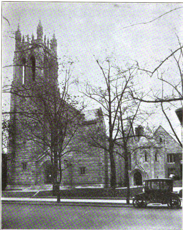
WASHINGTON CHURCH AND PARISH HOUSE.
