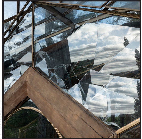
Image of the broken panels on Wayfarers Chapel due to the accelerated landslide
