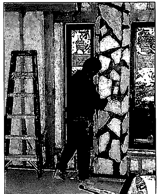
#9 - Wiring the rock: This close-up shows how the stone is wired to the form.
