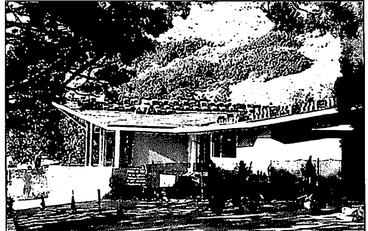
#7 - Tile roof: Cement tiles were loaded on the roof to "set" the framework for several days. After installation they were painted blue to match the Chapel roof tile.
