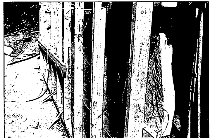
#9 - Wiring the rock: This close-up shows how the stone is wired to the form.
