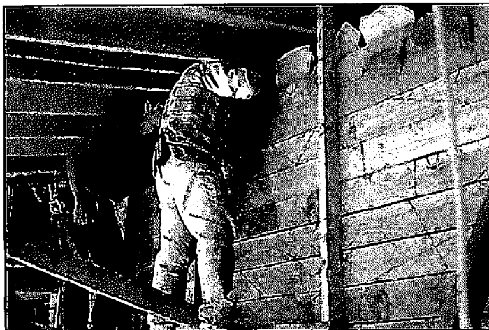
#11 - Lobby stone wall: The 12-foot high wall in the entrance lobby that will greet visitors is faced with stone. To complete the wall the cement had to be poured in from the top, a very difficult job. The stone mason found a piece of stone shaped like a heart that is now part of this wall.
