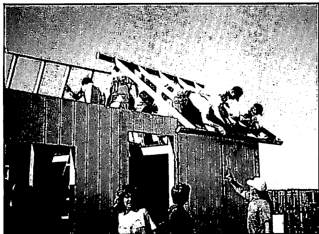
Securing the roof rafters.
