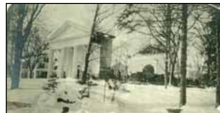
Low point for the Bath Temple: 1920 collapse from snow overload
