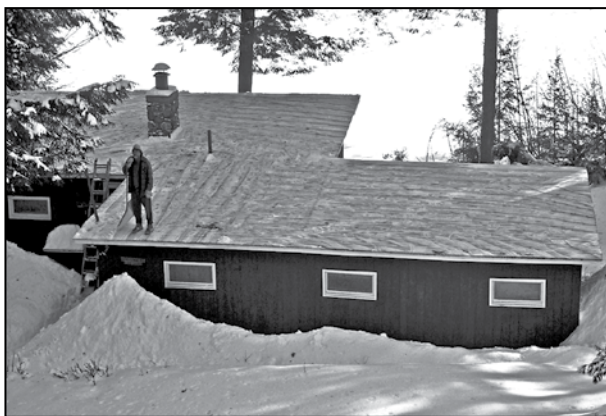
A winter's day—shoveling the roof
