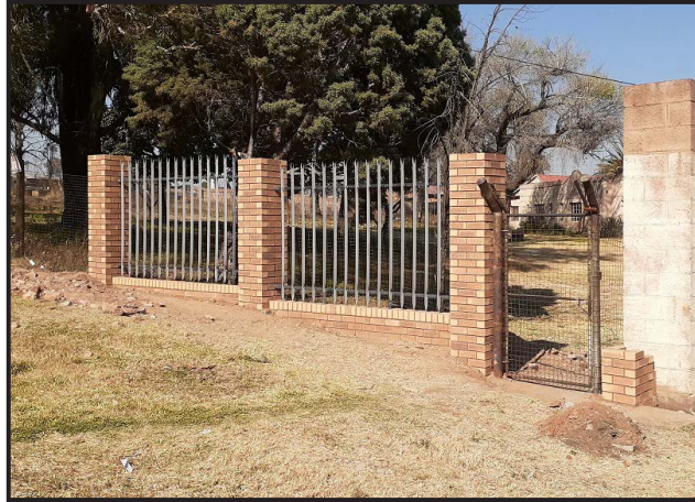
The beginning of the new wall around the church property, under construction.
