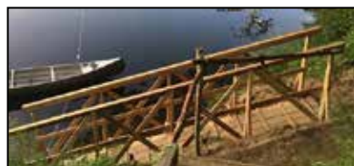
The new waterfront ramp
